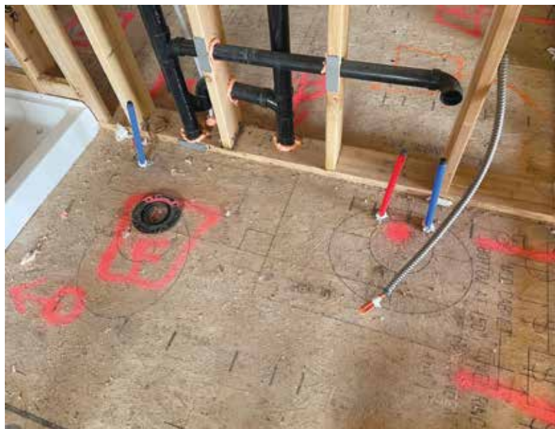
Above: Laser-engraved floor plan information depicting a typical bathroom layout. Below: Flashpoint's ILS (Integrated Layout System) showing laser-engraved plan information at a typical bathroom (black lines). Contractor used spray paint to perform further quality control following rough in.
