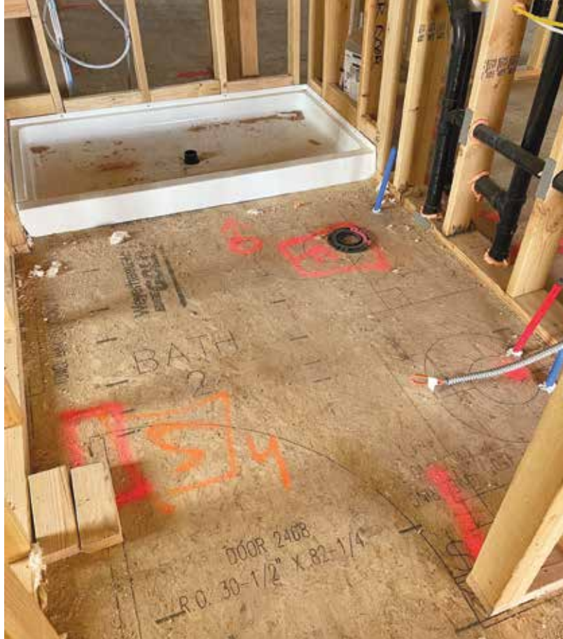
Above: Laser-engraved floor plan information depicting a typical bathroom layout. Below: Flashpoint's ILS (Integrated Layout System) showing laser-engraved plan information at a typical bathroom (black lines). Contractor used spray paint to perform further quality control following rough in.
