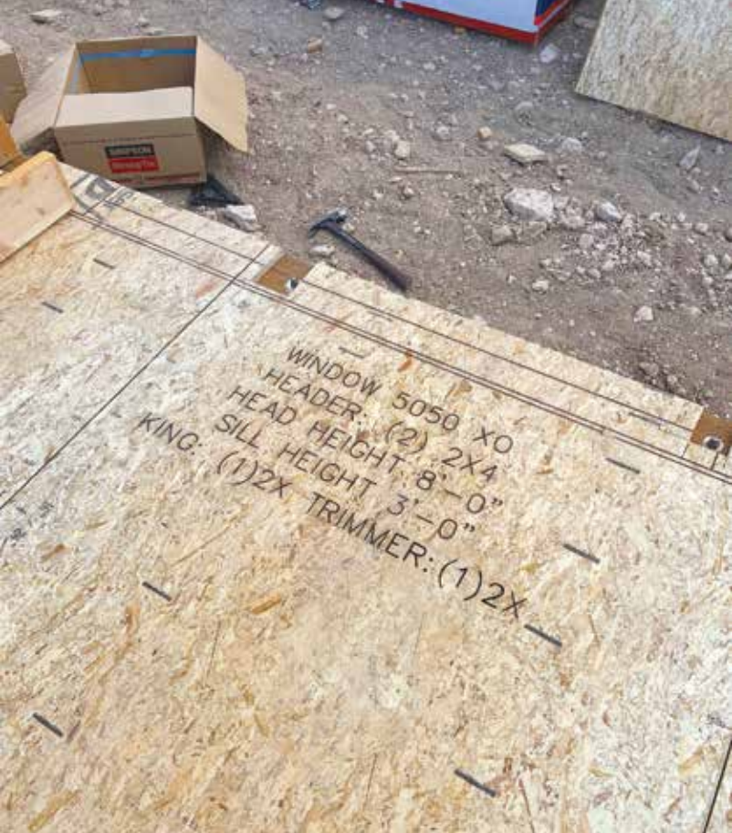
Information from the original plan set consolidated into one comprehensive note depicting how and where to build a window opening.
