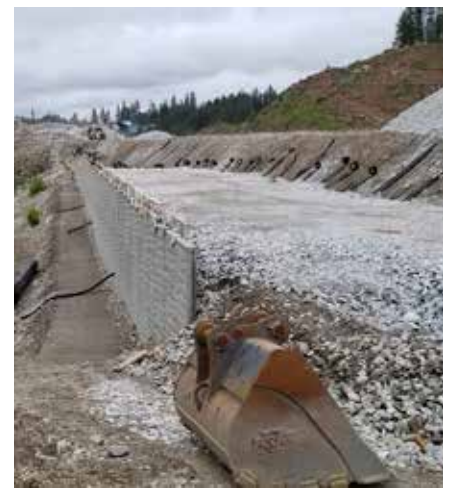
Construction of mechanically stabilized earth (MSE) Wall
