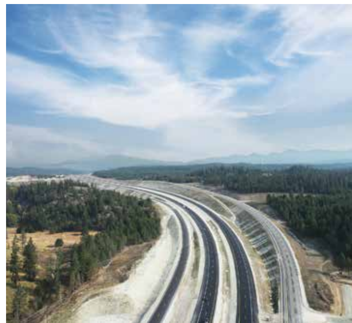
US-95 looking north. Completed project photo. From left to right: Vintage 95 Road, southbound US-95, northbound US-95, and Mineral Ridge Road.
