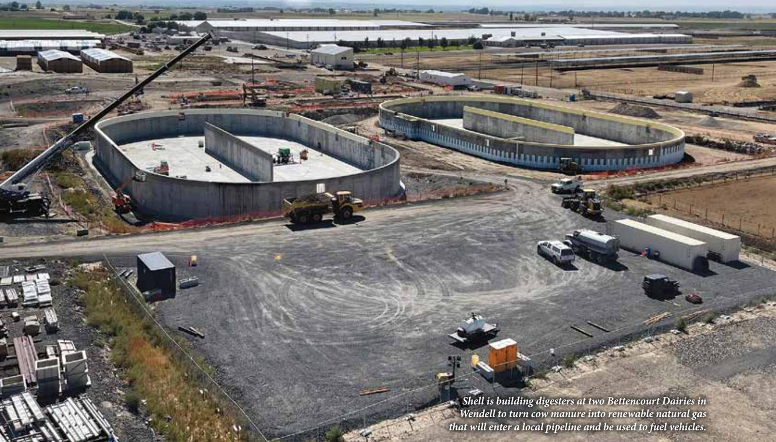
*Shell is building digesters at two Bettencourt Dairies in Wendell to turn cow manure into renewable natural gas that will enter a local pipeline and be used to fuel vehicles.*
