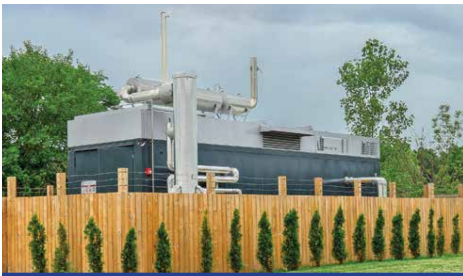
The City of Windsor in Ontario, Canada, recently installed a combined heating and power system at its Huron Lodge care facility, a 177,000-square-foot, long-term care home for all ages that is one of the largest consumers of gas and electricity in the municipality.
