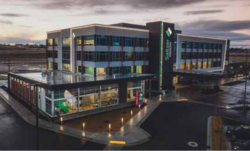
Saltzer Health worked with Ball Ventures Ahlquist to construct this new medical office building on 10 Mile Road in Meridian. The building houses Idaho's first 24-hour urgent care clinic. IMAGE COURTESY OF SALTZER HEALTH.
