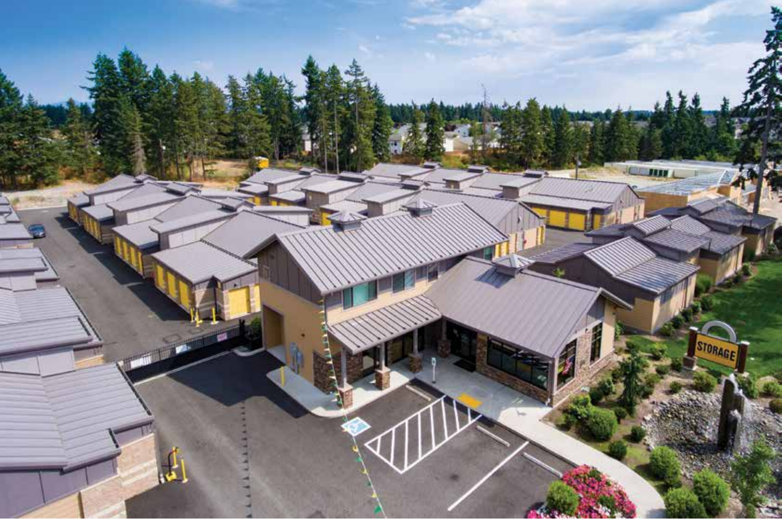
North Graham Storage.
